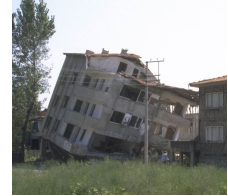
Fig. 1: Building damage induced by seismic loading.
